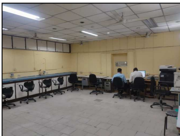
ARIS Lab-cum-Server Room
